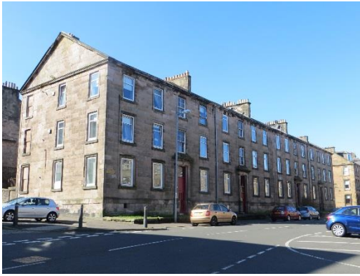
Figure 25 Windows replaced in uPVC
