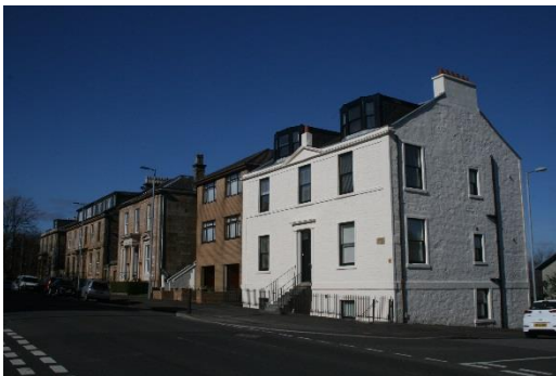
Figure 23 Painted stone walls
