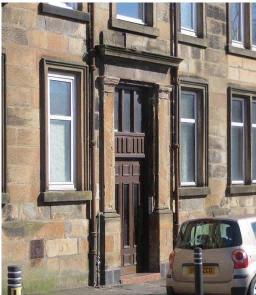
Figure 24 Cement-based repairs
