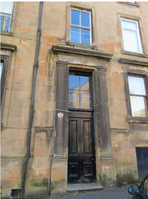
Figure 16 Timber windows, and door with rectangular lay light
