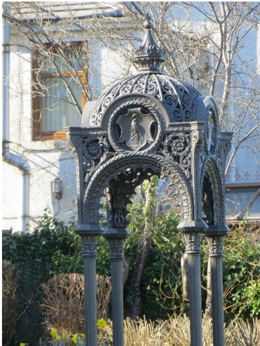
Figure 19 Cast iron canopy
